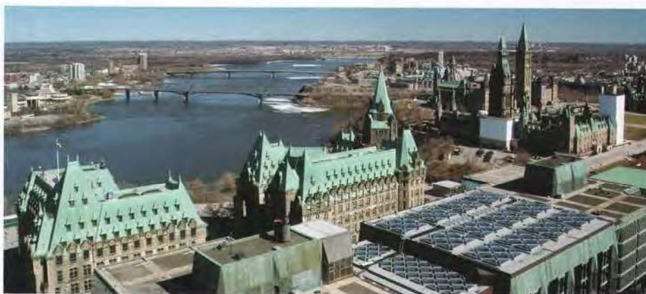
Figure 1 A colorful patina develops on copper roofs over several years
