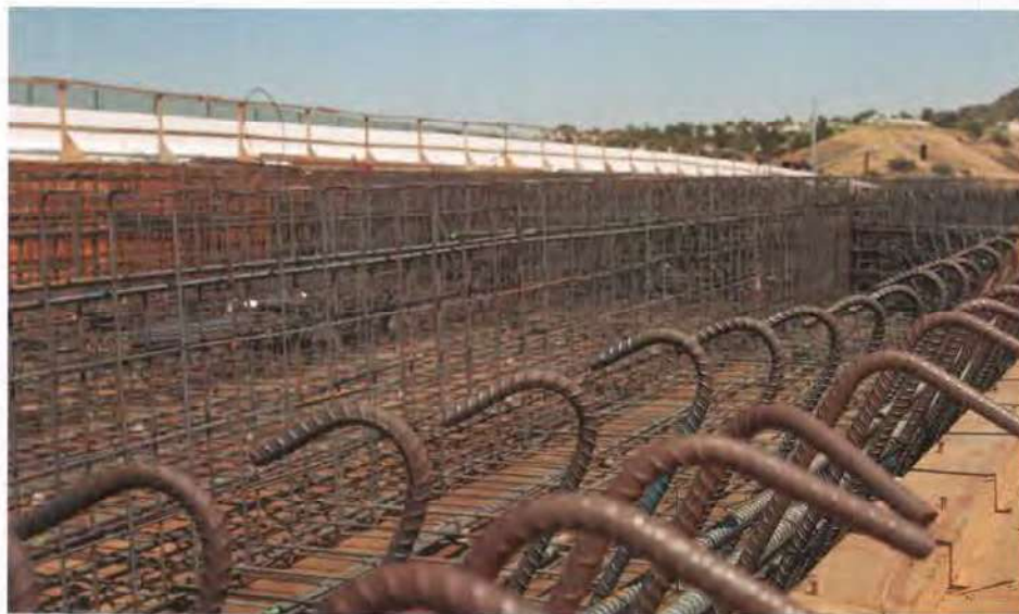
Figure 4 Galvanized steel is corrosion resistant and requires no maintenance.
